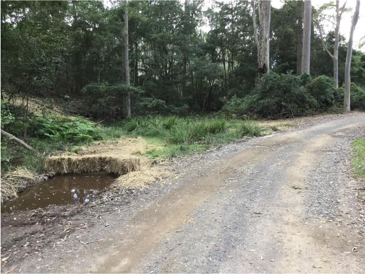
Figure 12 - northern approach to crossing 2 showing cleaned silt pond and haybales.
