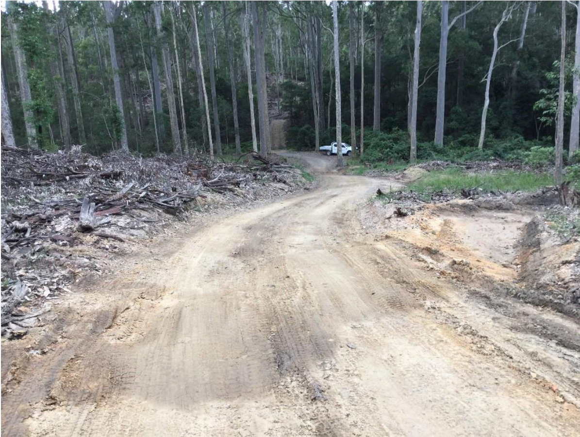
Figure 8 – example of newly installed extended mitre drains on Cpt 3058/5 Rd, southern approach of crossing 2
