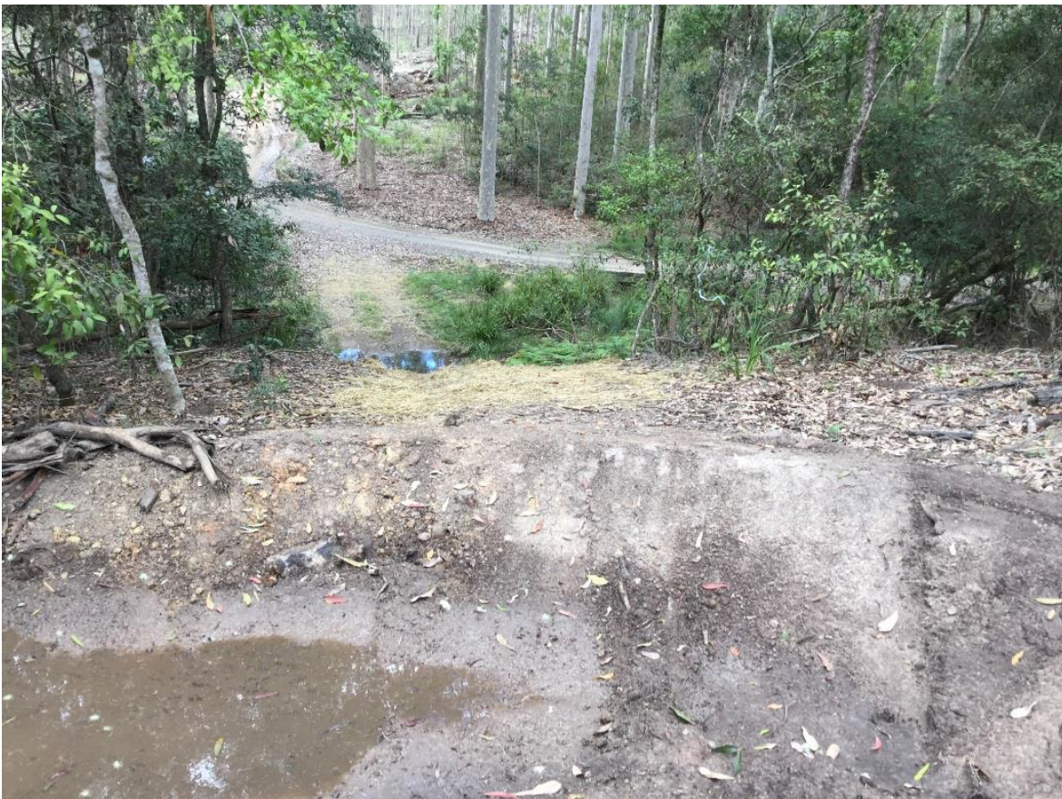
Figure 11 - old track, looking south over newly installed rollover drain.
