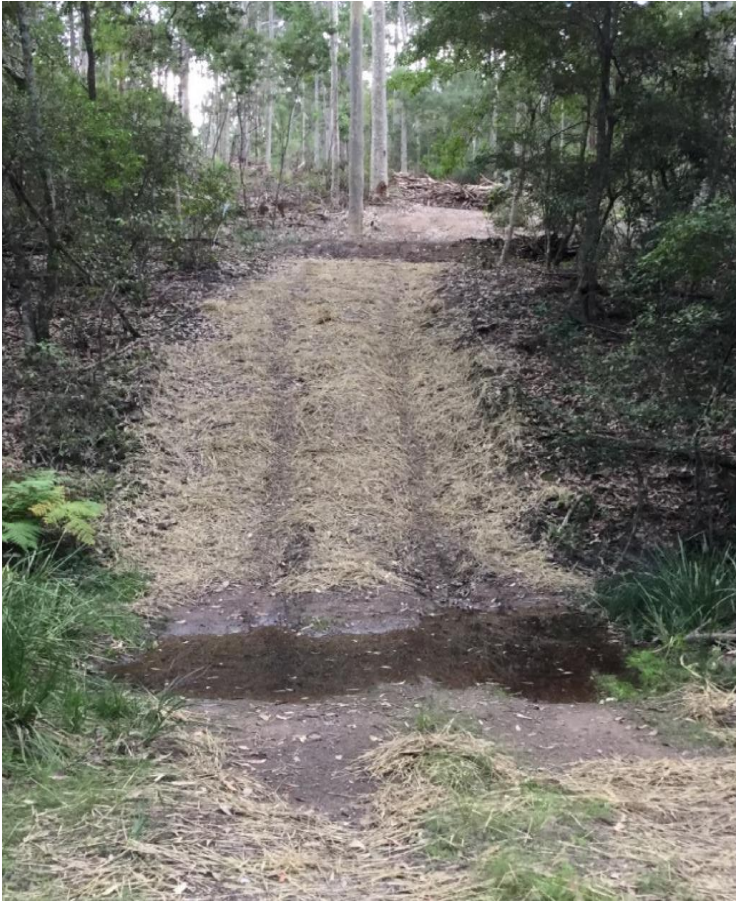
Figure 10 - old track, looking north, showing seed and mulch and rollover drain at 20m.
