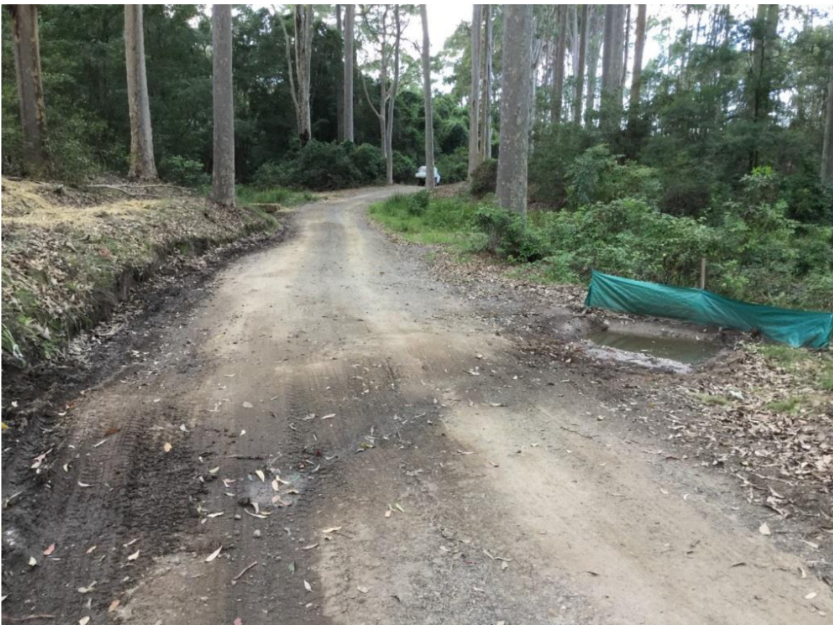
Figure 7 - new extended mitre drain, cleaned sediment pond and repaired silt fence on northern approach of crossing 2.
