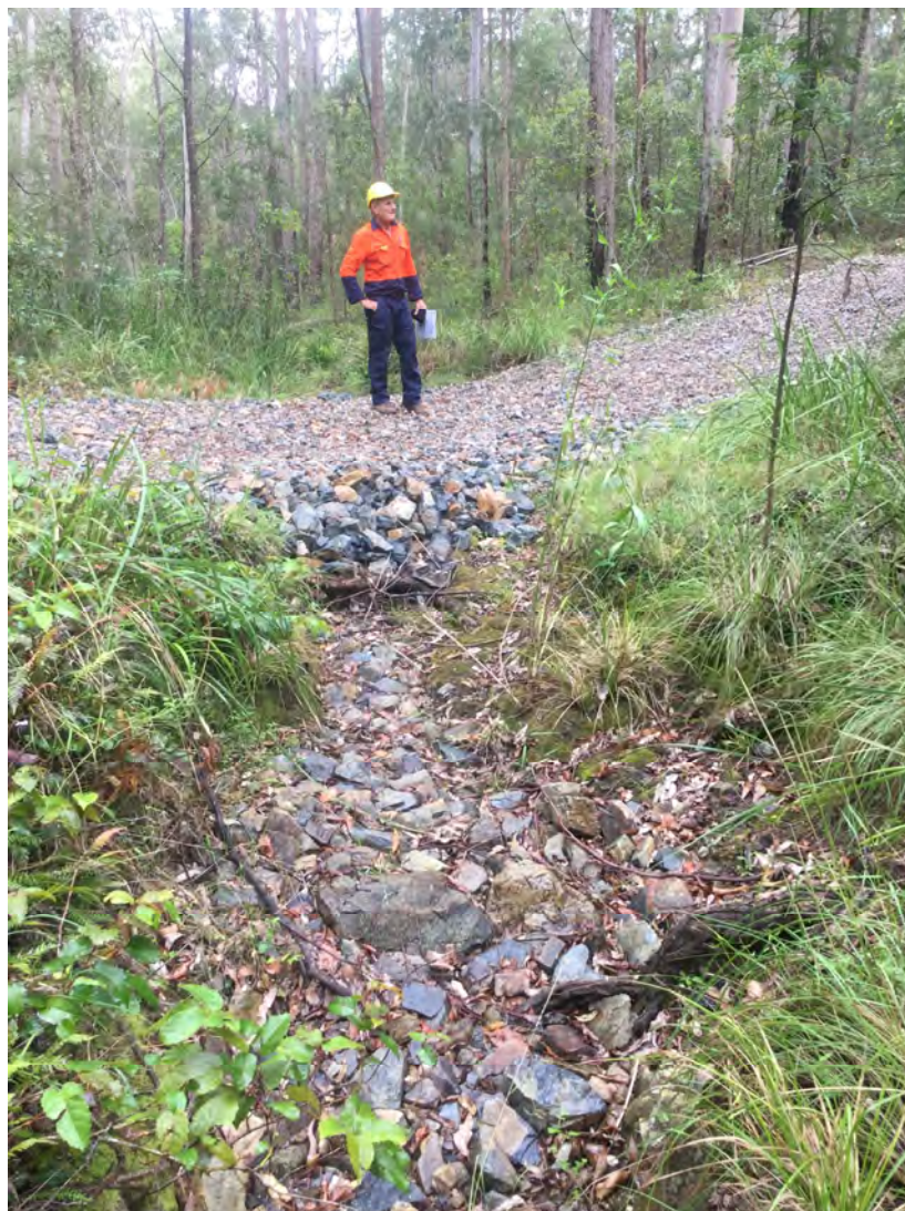
Figure 14. Upstream approach of Crossing B, raised above channel.
