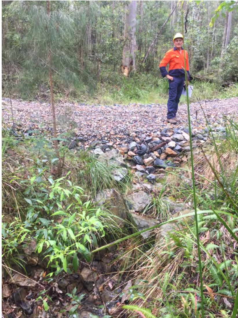
Figure 15. Downstream edge of Crossing B, smaller rocks exposed along edge and causeway raised above channel. Inadequate containment of crossing surface reducing ability to withstand high stream flows.
