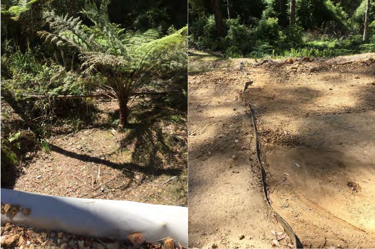
Photos 12: stream bed of 3 rd order stream with no pollution. Photo 13: Rubber strip drainage starting to fail.
