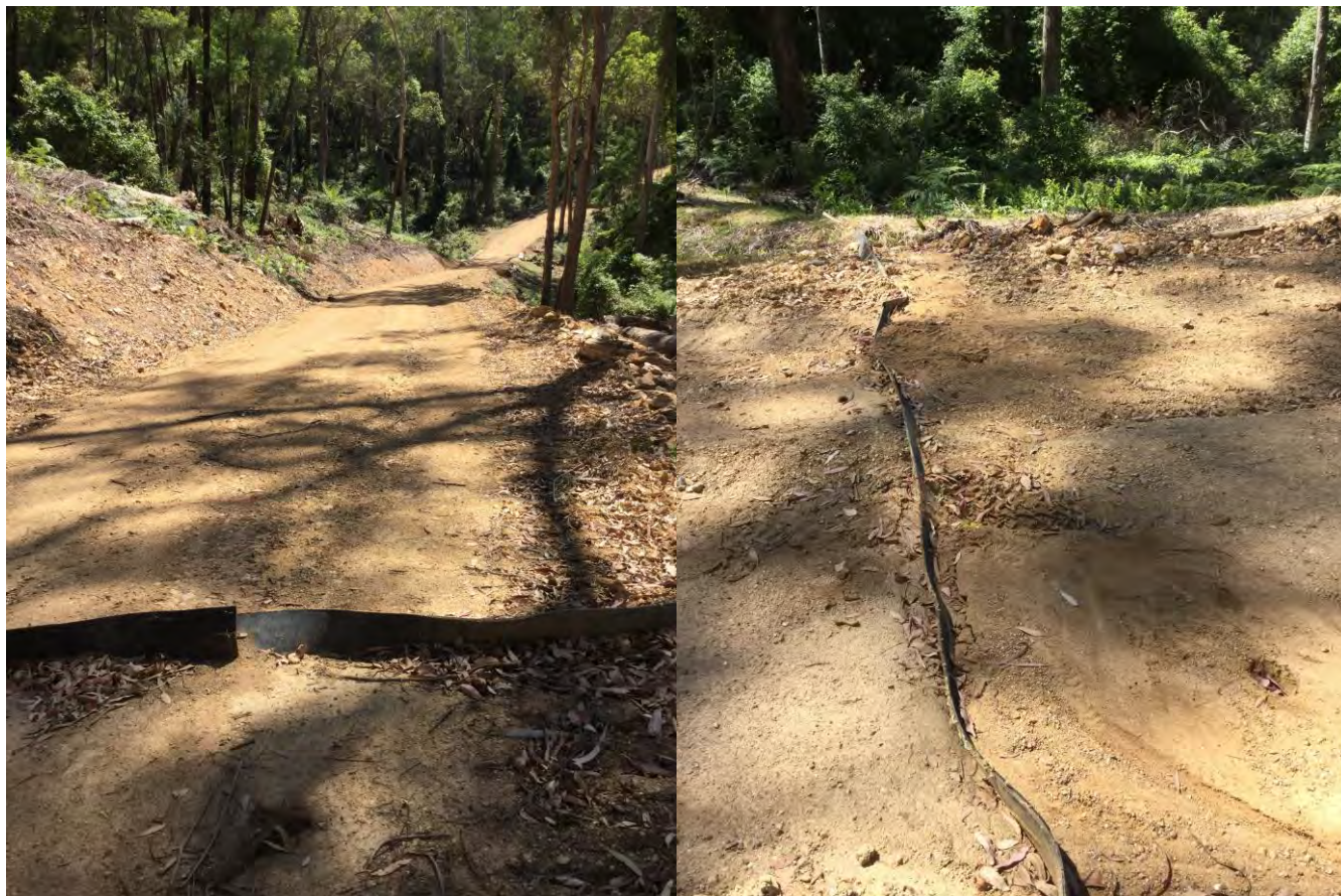
Photos 8 & 9: Problematic rubber strips used as drainage structures on crossing C1
