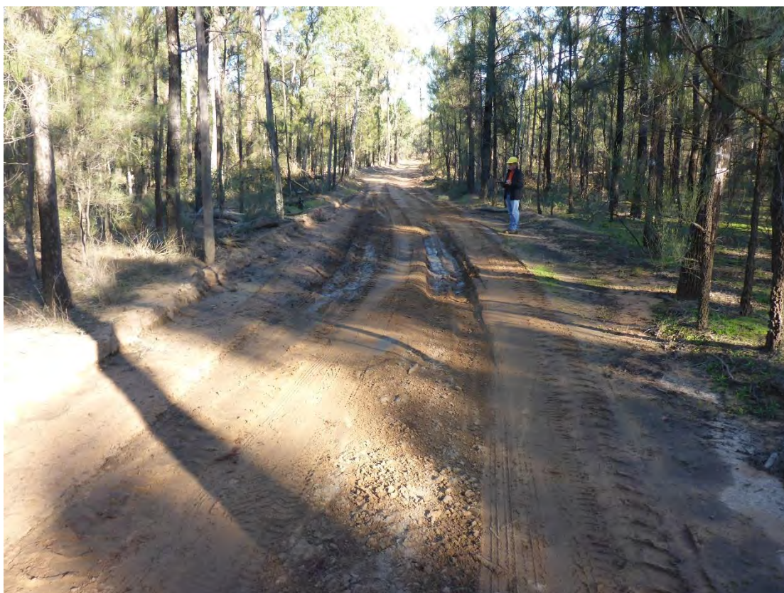
Photo 75, Wpt 1 – Unstable natural surface crossing of drainage depression. View from centre of crossing looking west.
